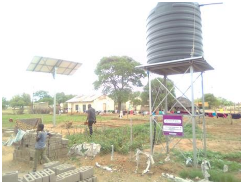
St Francis of Assisi Anglican Church, Tsholotsho, with the Solar Installation
