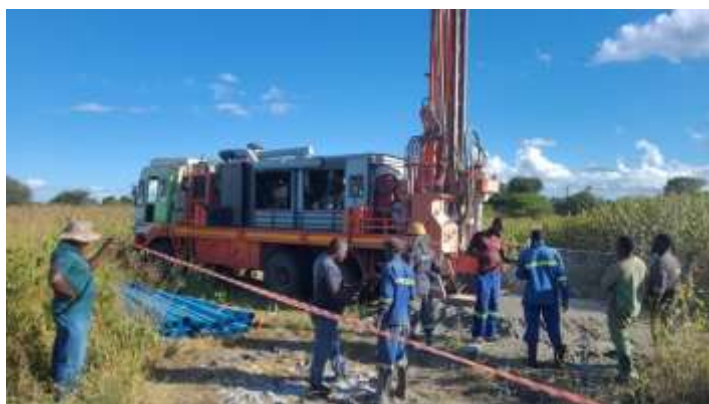
4: The Drilling Rig arrives on Site
